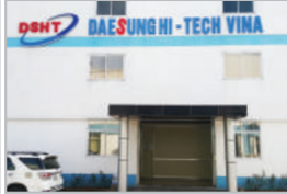
Vietnam DAESUNG HI-TECH VINA TS9 Street, Tien Son Industrial Zone, Tuong Giang Commune, Tu Son Town, Bac Ninh Province
